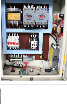
No. 3 Electric Cabinet
